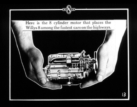
Mere are a few things wor-Lefthy of your consideration Eight cylinders, 31/8 ×4", Full Pressure Feed Lubrication. Balanced and Counterbalanced Crankshaft, Vibration Dampener, Rubber Engine Mounting.
