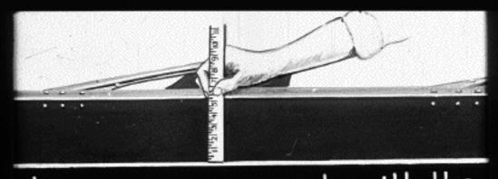
Impress your prospects with the unusually strong Willys frame. It is 51/4 inches deep with 6 heavy cross members riveted to both upper and lower flanges of side rails.
